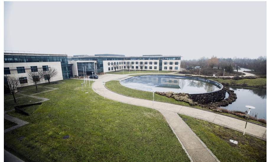
→ SAFRAN Advanced Casting Research Center under construction at Gennevilliers ▪ state-of-the art facility covering the whole turbine blade manufacturing process
